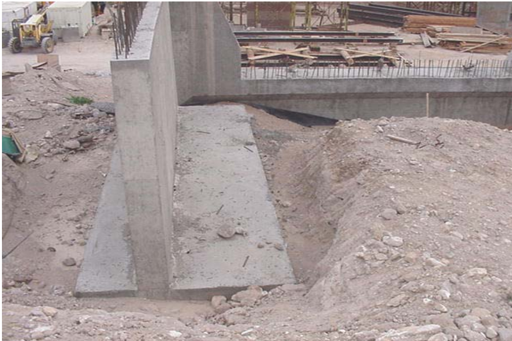
Figure 8-5. Abutment/wingwall footing, I-10, Arizona.
